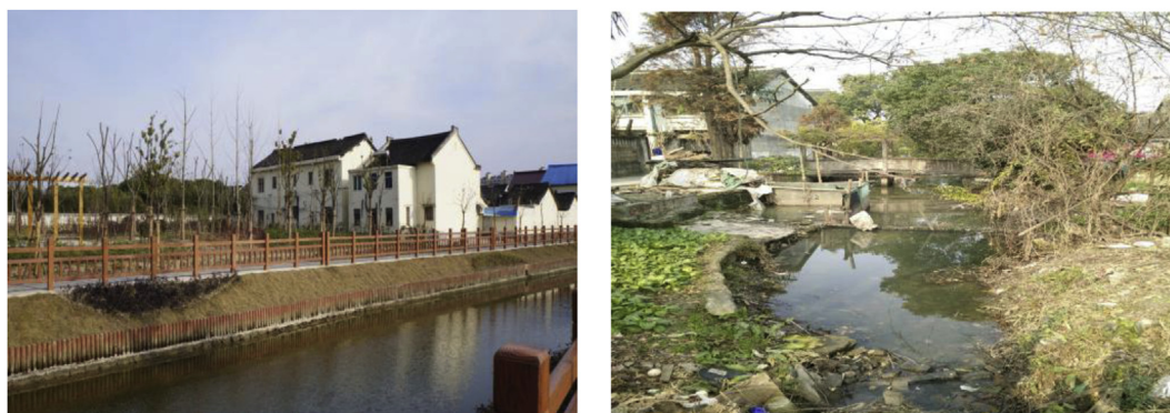
Fig. 4. Comparison of river conditions between Heping Village (left) and Tangwan Village (right). Sources: authors' photos.
